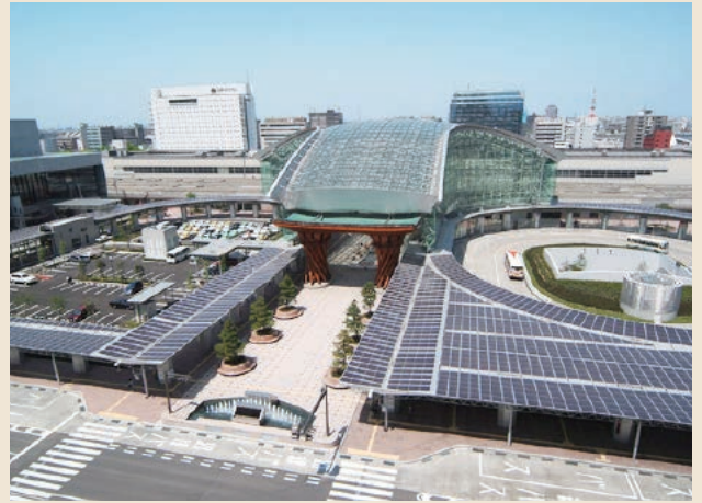
JR Kanazawa Motenashi Dome (above ground)
